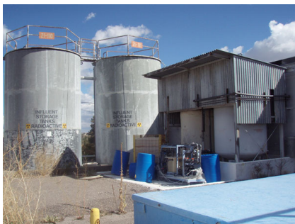
Building and structures to be decontaminated and demolished
