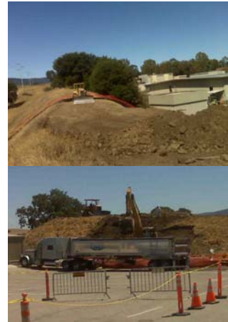
Artificial Ridge excavation
