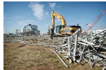
D&D of an Idaho Site building
