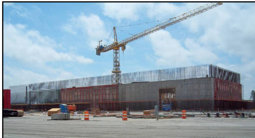
MOX Facility Construction at SRS
